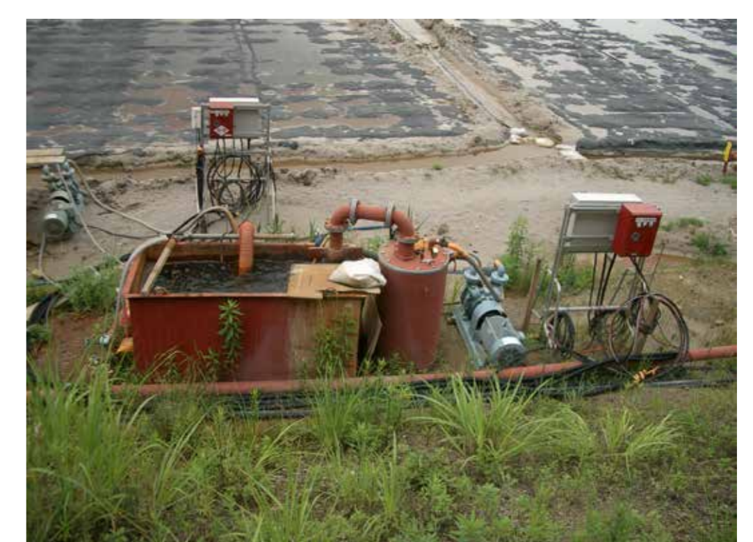
6 Apply Suction Vacuum pump
