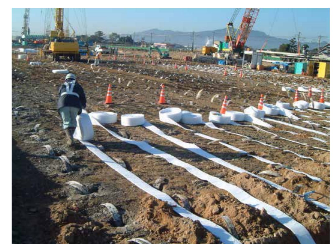
3 Spreading Horizontal Drains
