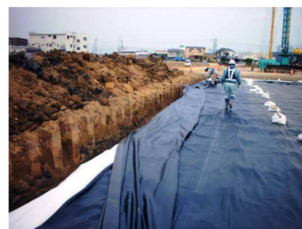
4 Spreading Airtight sheet
