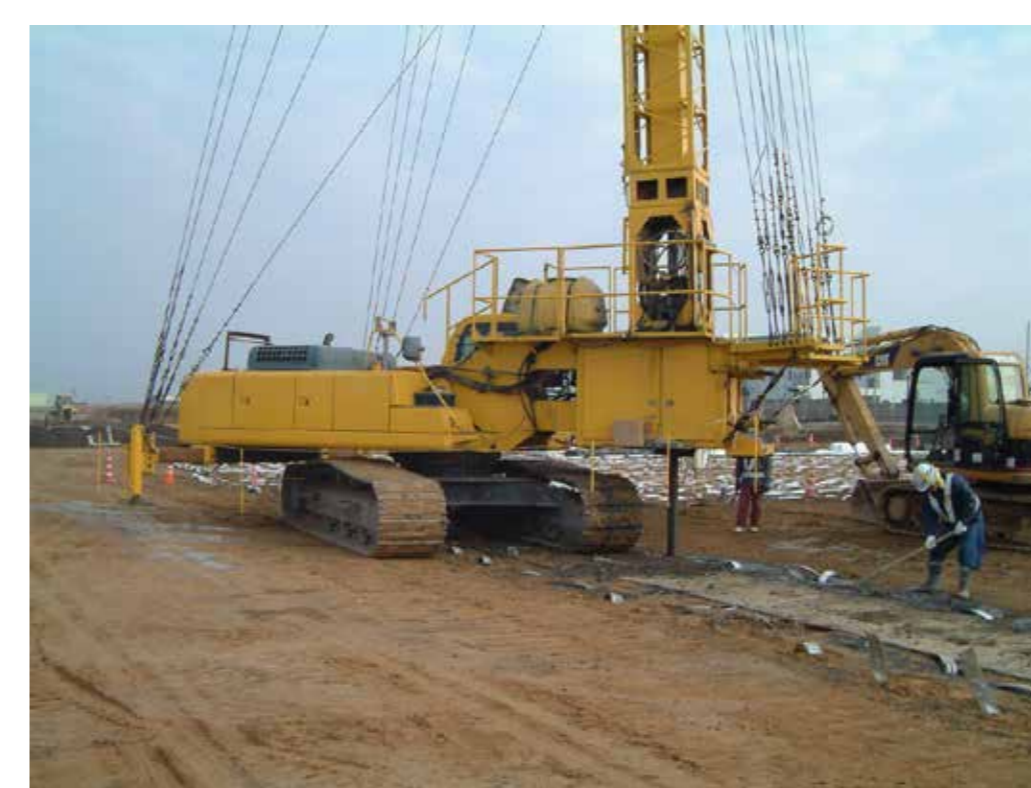
1 Installation of Vertical Drains
