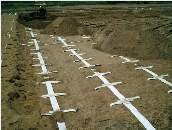
(Picture shows experimental comparison between sand mat and SB Drain in the East-West highway Vietnam project.)
