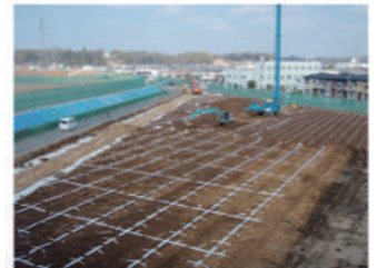
PVD ground improvement
